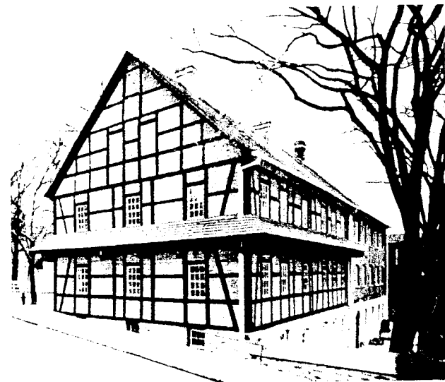
Single Brothers' House (1769), Salem, N.C., a Moravian Fachwerk building extended by a brick addition in 1786. (Old Salem, Inc.)
