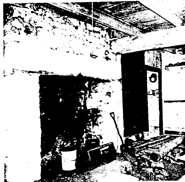
Kitchen of the Philip Dellinger House (c. 1815), Shenandoah County, Va. The exposed ceiling framing, masonry fireplace and log walls are typical of German immigrants' tendency to express individual building parts.
