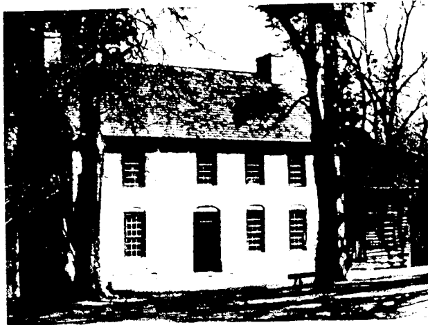
Michael Braun House, Rowan County, N.C., an example showing changes in building design resulting from late 18th-century acculturation
