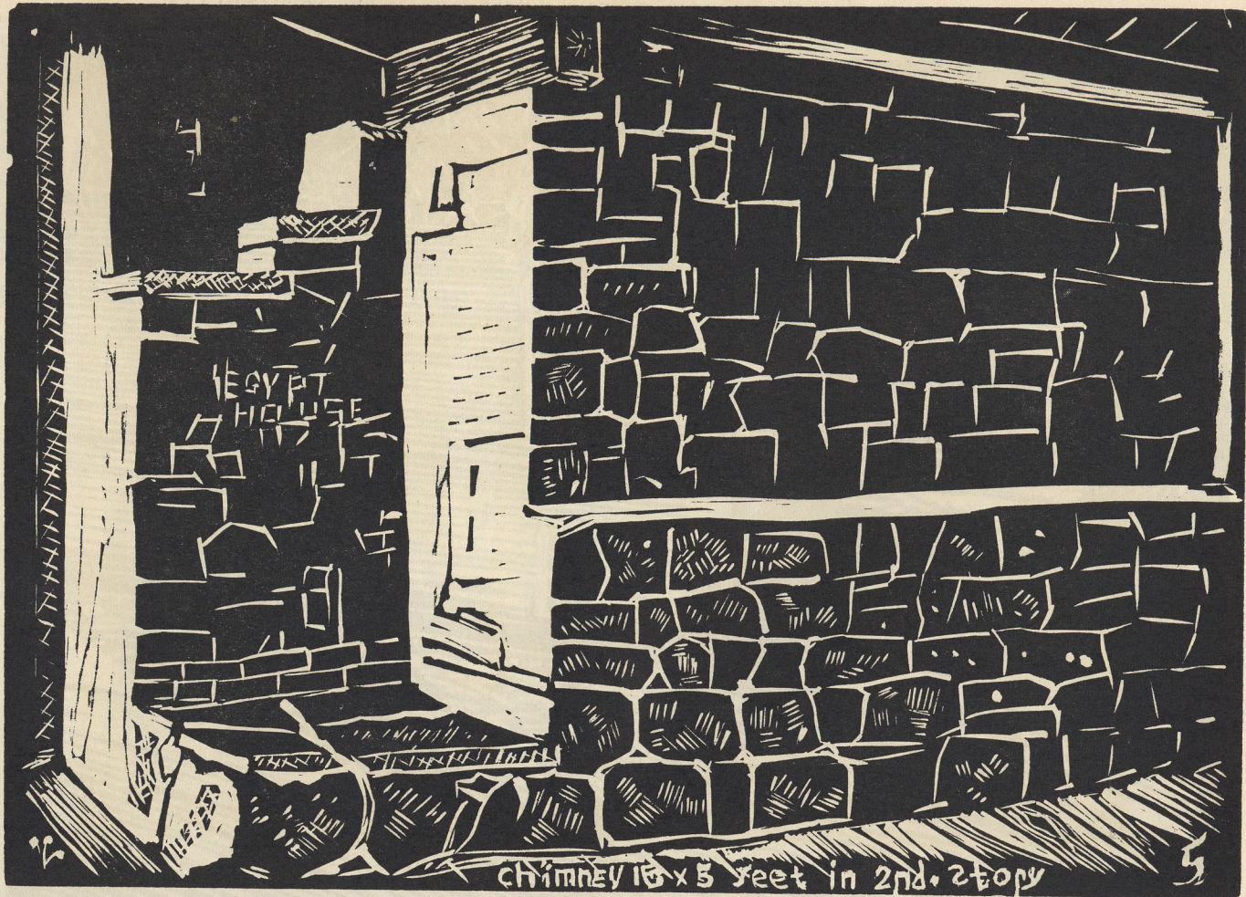
CHIMNEY IN THE CENTER OF EGYPT HOUSE, 15 by 5 feet in second story. Files of the Historic American Buildings Survey contains eleven large sheets or designs of this house under title of "Fort Egypt."
